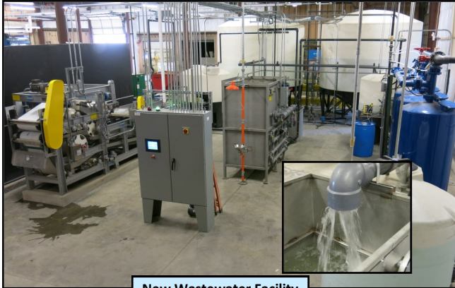
New Wastewater Facility
