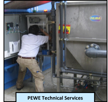
PEWE Technical Services Installation Start-up Support
