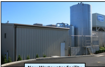
New Wastewater Facility
