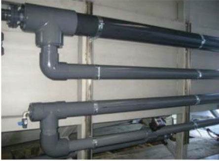
From left to right: If space is a premium, Coagulants and flocc agents can be added within the piping manifold. Note the sampling ports added in this one. Next, a sloped bottom design makes removing settling solids much easier. The photo on the right shows a liquid solids separation system designed and built by P.E.W.E.
